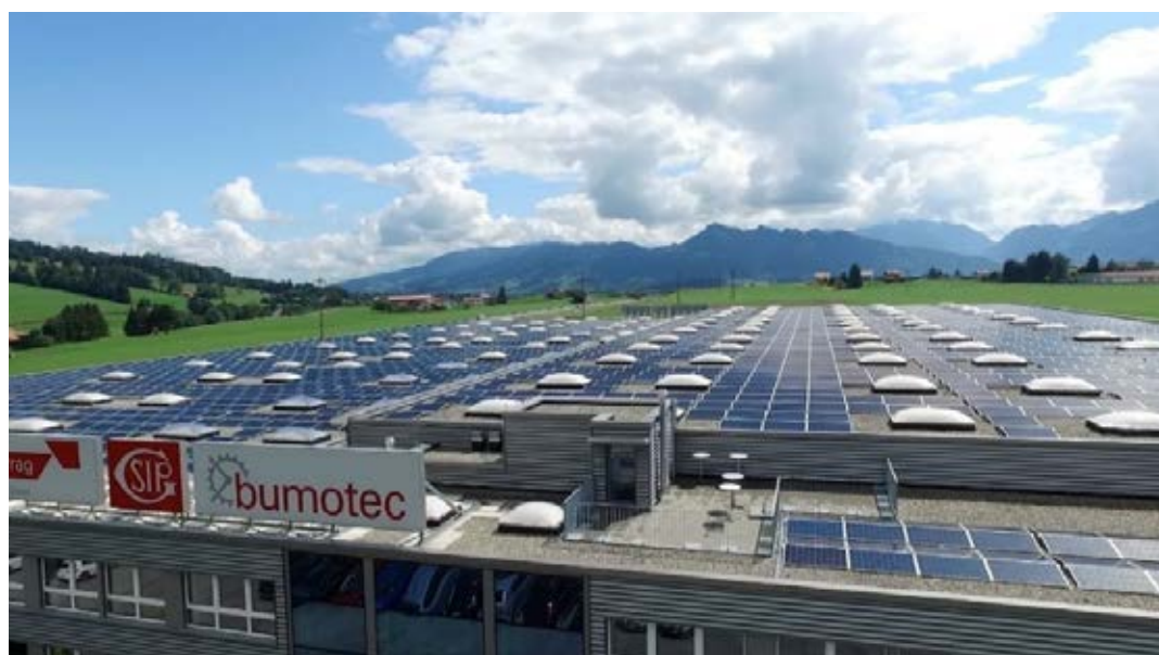
Solar installation on our manufacturing plant in Vuadens, Switzerland, that covers about 40% of the local electricity consumption
